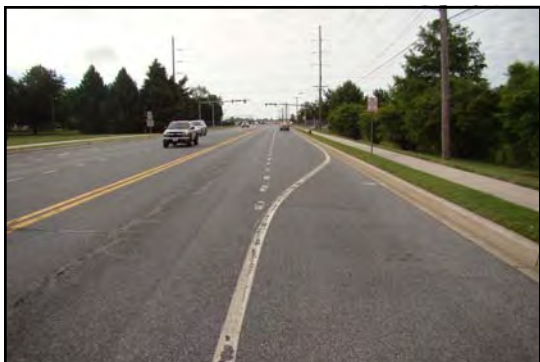
Saulsbury Road /Gateway Boulevard
